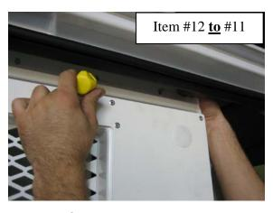
Align 3<sup>rd</sup> Compartment Doorframe to 3<sup>rd</sup> Compartment Ceiling and loosely attach 1/4" x 3/4" hex head bolts, washers and serrated nuts.
